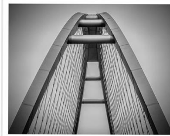
TG-1218 | The Underpass
